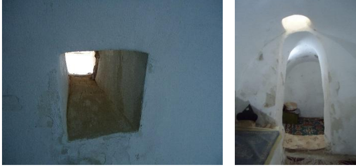
Figure 10a. Side ventilation chimney (Author - 2021)
