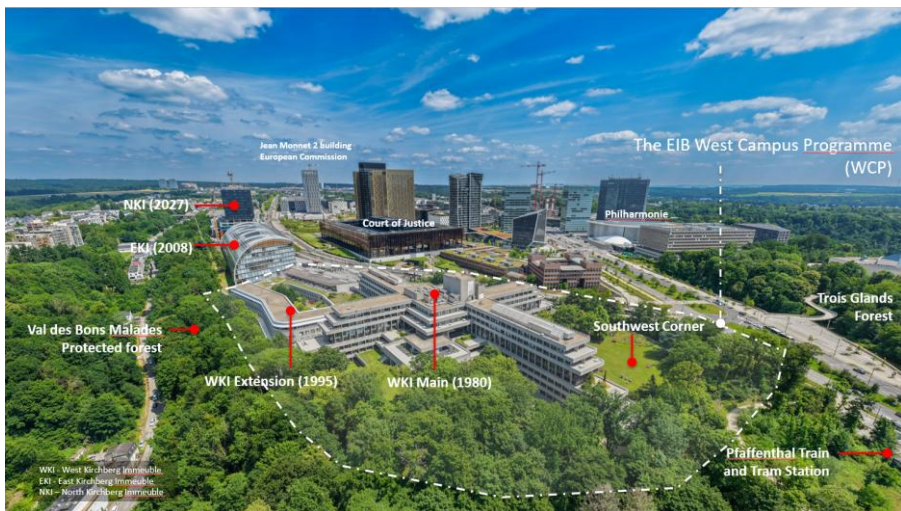
Figure 1: Drone view of the WCP area looking eastwards.
