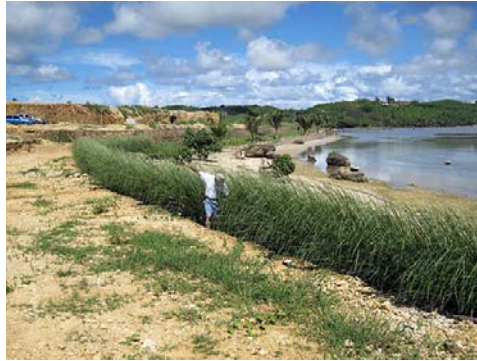
Plate 4. Vetiver grown along river bank mitigates flood damage by dissipating the energy of the water flow to the community.
