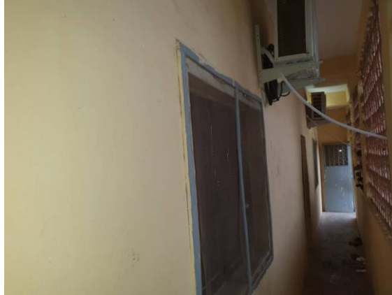
Fig.10: Showing the corridor, the Inverter Air Conditioner, the solar shading bricks, windows and enough lighting during the day (Field Survey, 2020).
