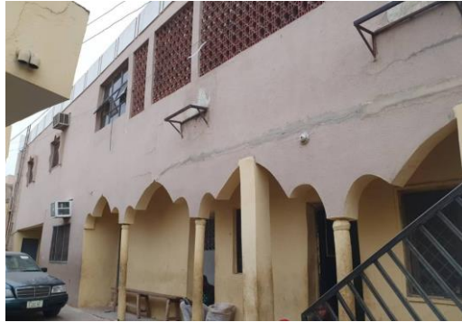
Fig. 6 Showing the arrangement of windows and solar shading red bricks in the green building (Field Survey, 2020).
