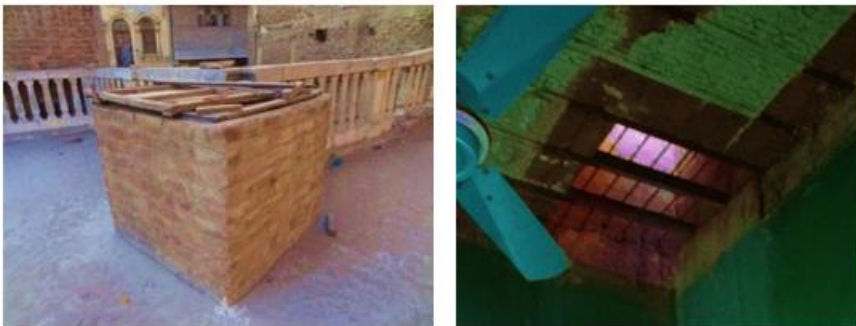
Figure 15: Wind Chimney for cross ventilation
