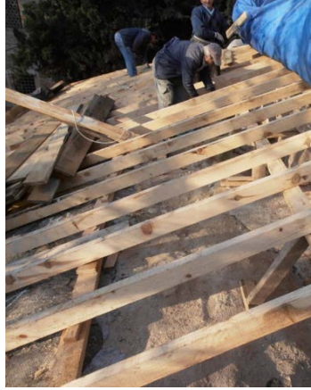
Figure 2. Restoring the vaults of Murat II. Tomb Roof
