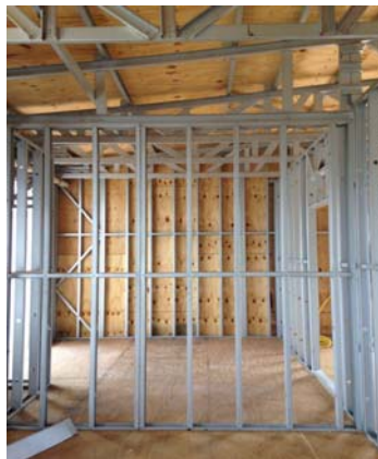
Image 2: Light Steel Framing housing construction site (Authors)
