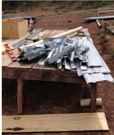
Image 3: Total waste in a Light Steel Framing construction site (Authors)
