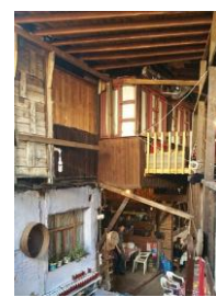
Figure 21. The open anteroom is closed due to annex (Source: the Authors)
