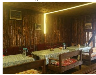
Figure 19. New wooden siding on the masonry walls of ground floor (Source: the Authors)
