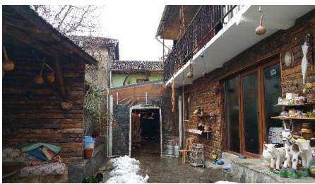
Figure 8. New reinforced concrete building in the backyard (Source: the Authors)
