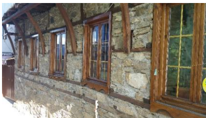
Figure 14. New openings on the ground floor walls (Source: the Authors)
